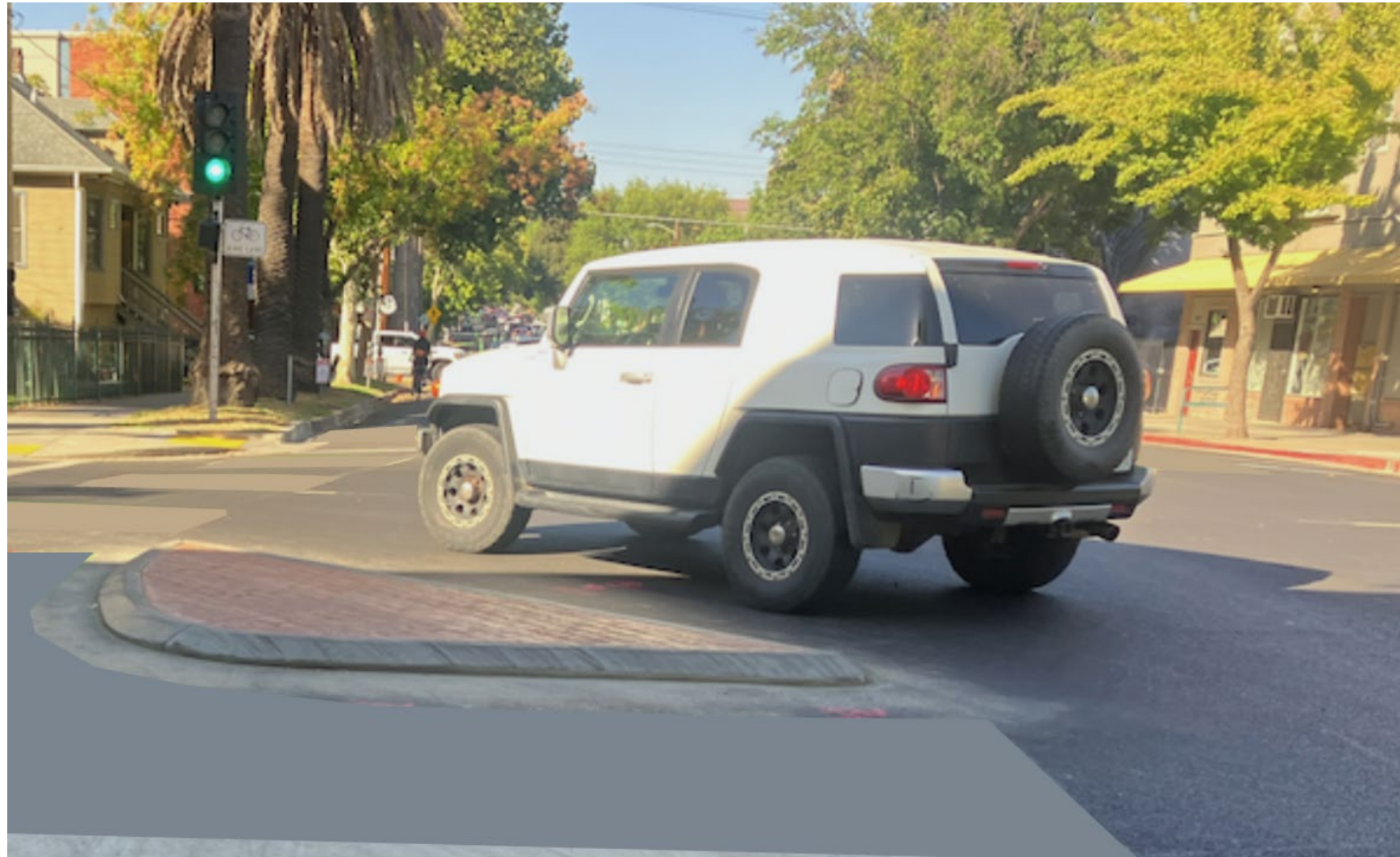
Sample of Mountable Corner Islands for Protected Intersections. Source: NACTO
