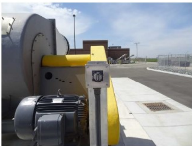
Figure 15.4: Biofilter Fan HOA Selector Switch.
