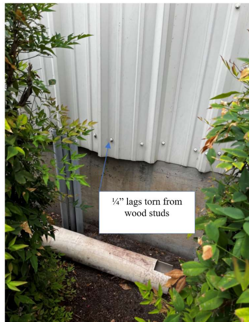
Buckling of Siding Due to Settlement
