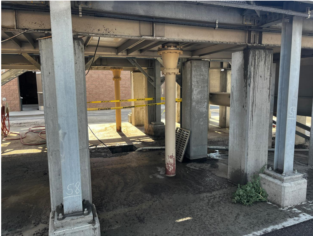
Figure 17 Screen Manhole Under Screw Presses – Location of Overflows
