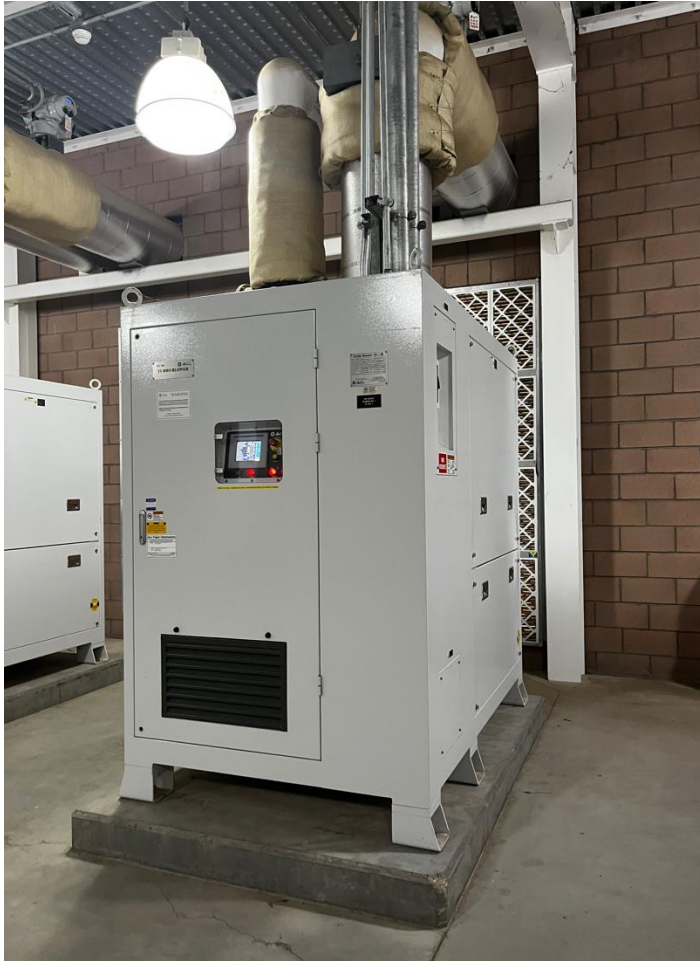
Figure 10 Air Scour Blower No. 1
