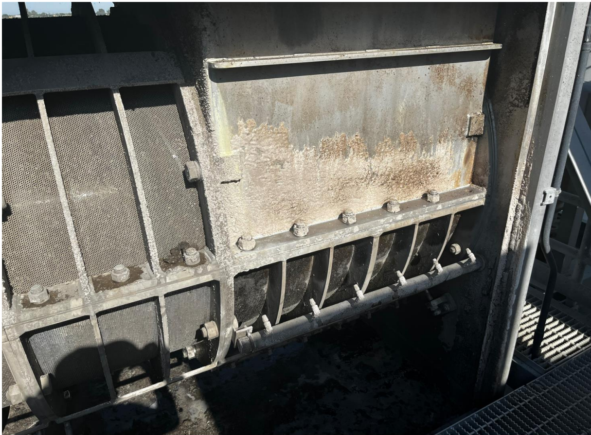
Figure 16 Struvite Formation on the Screw Press
