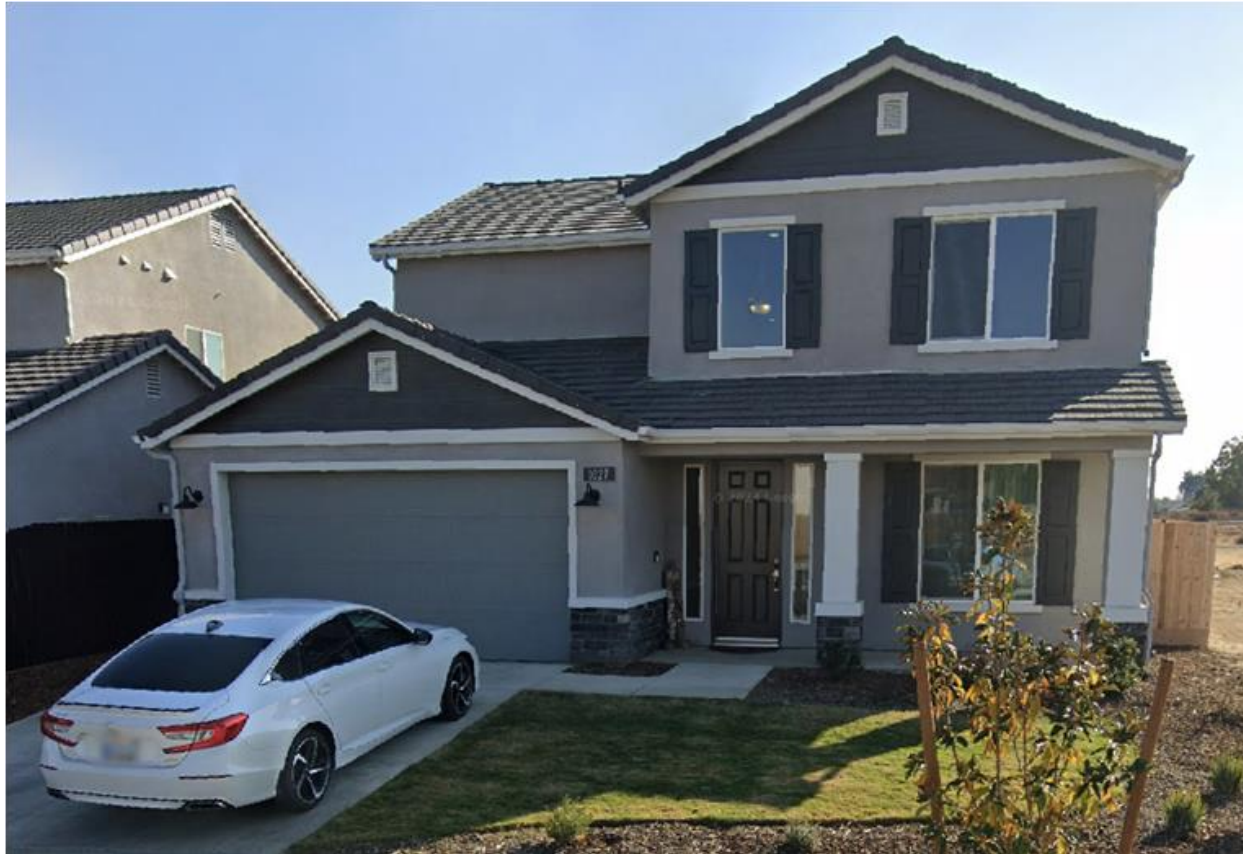
1215 E. Seeger Court – Morgan Enterprises Construction
