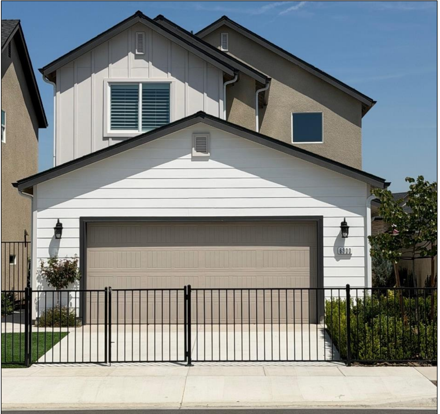
Exhibit 3. The front elevation of this model home in Goshen has no ground floor windows and the front door faces the side yard fence, resulting in an absence of “eyes on the street”. The garage dominates the front of this house to the degree that one would not unreasonable to assume this is the back of a house facing an alley.
