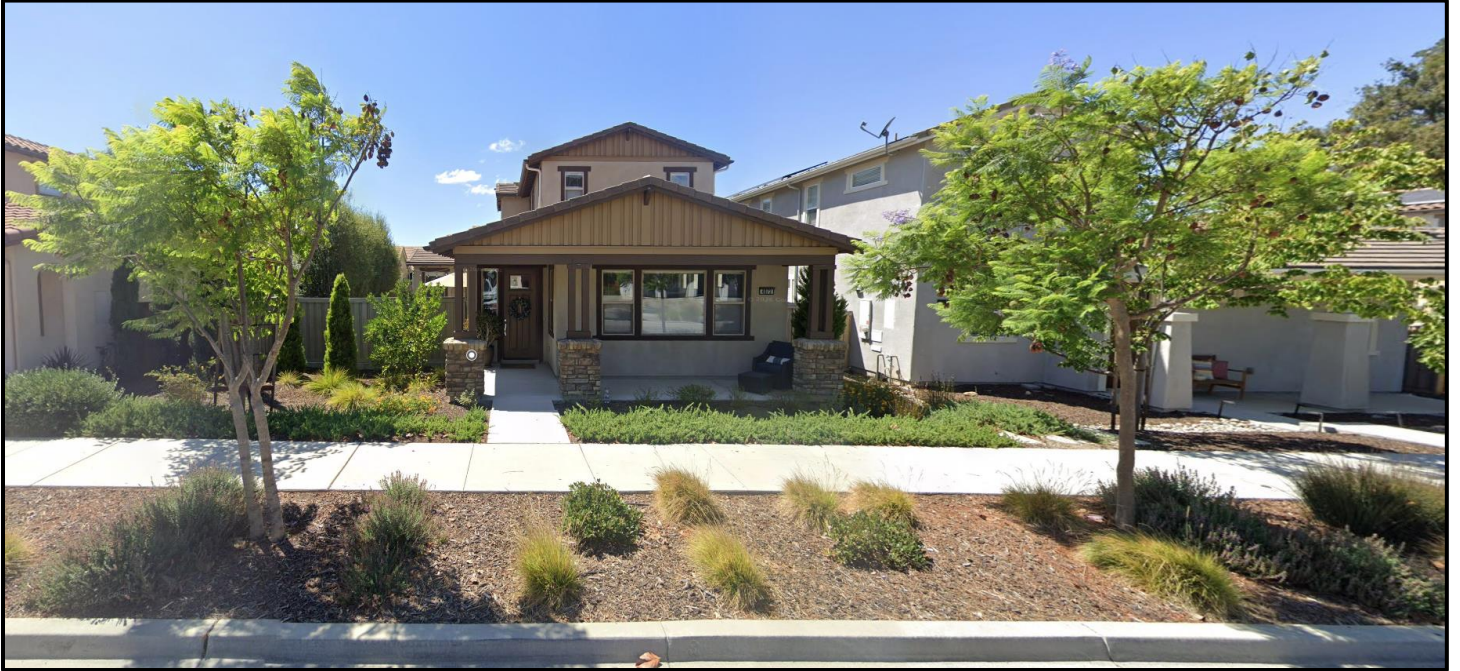
Exhibit 10. A view of the front of the alley-loaded homes shown above. A lack of driveways along the front of the house allows for increased street tree density.
