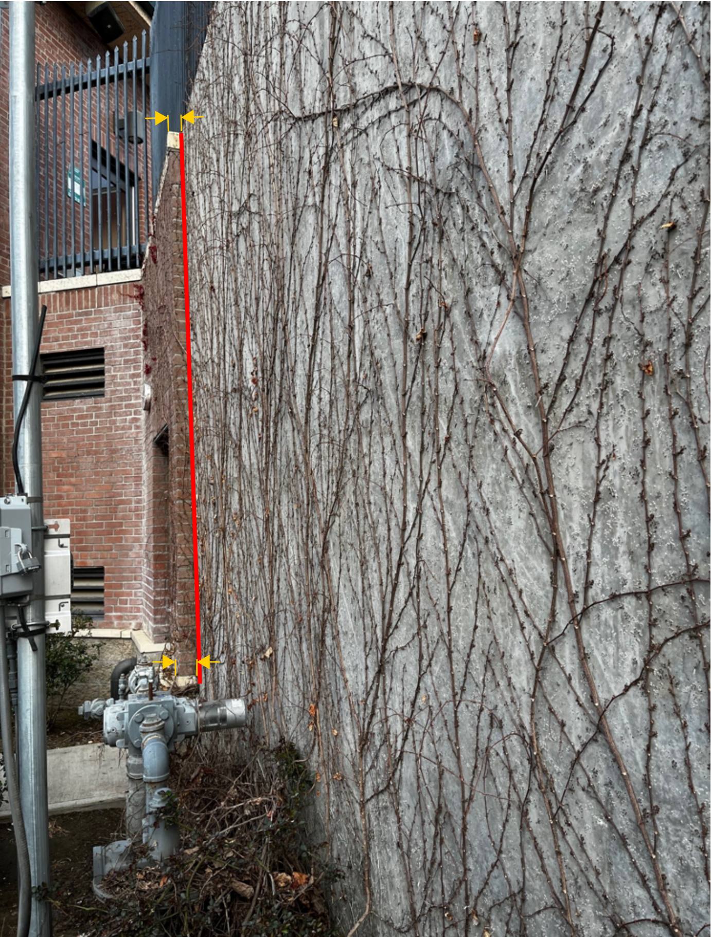
Pic.1 - Retaining wall in comparison to the adjacent brick showing the tilt in the wall. The yellow arrows show the visible brick at the top vs. the bottom. The leaning of the wall has caused more coverage of the brick at the top of the wall.
