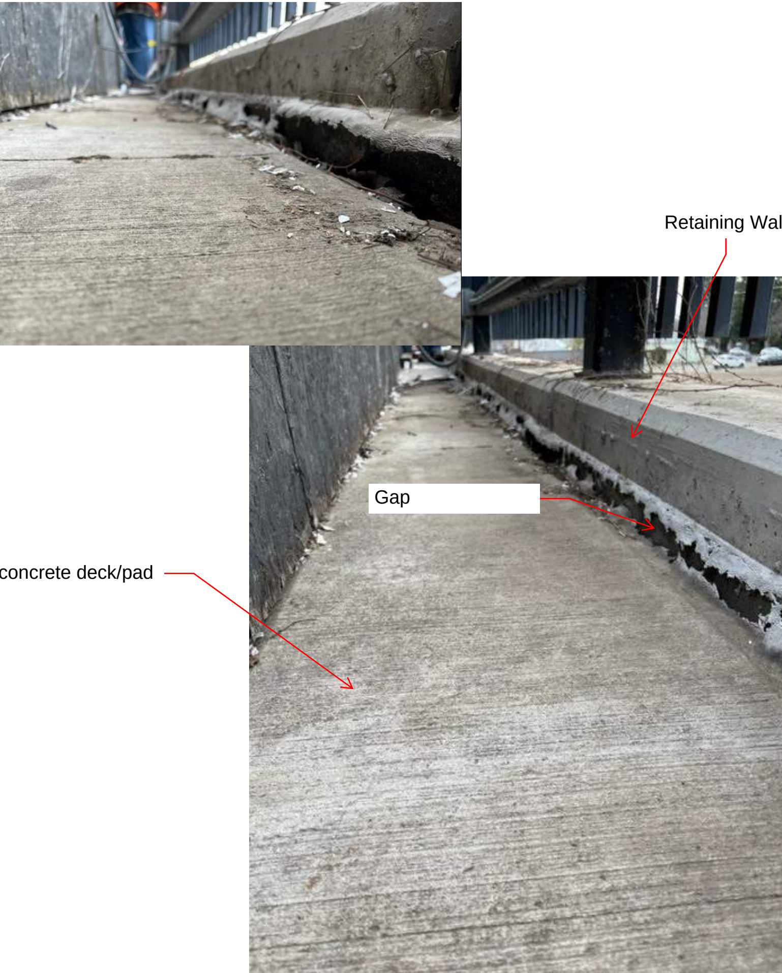
Pic. 3/4 - Gap Between upper Concrete Pad/Deck and the Retaining wall
