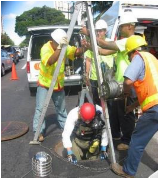
Photo 2-1. Confined Space Entry
