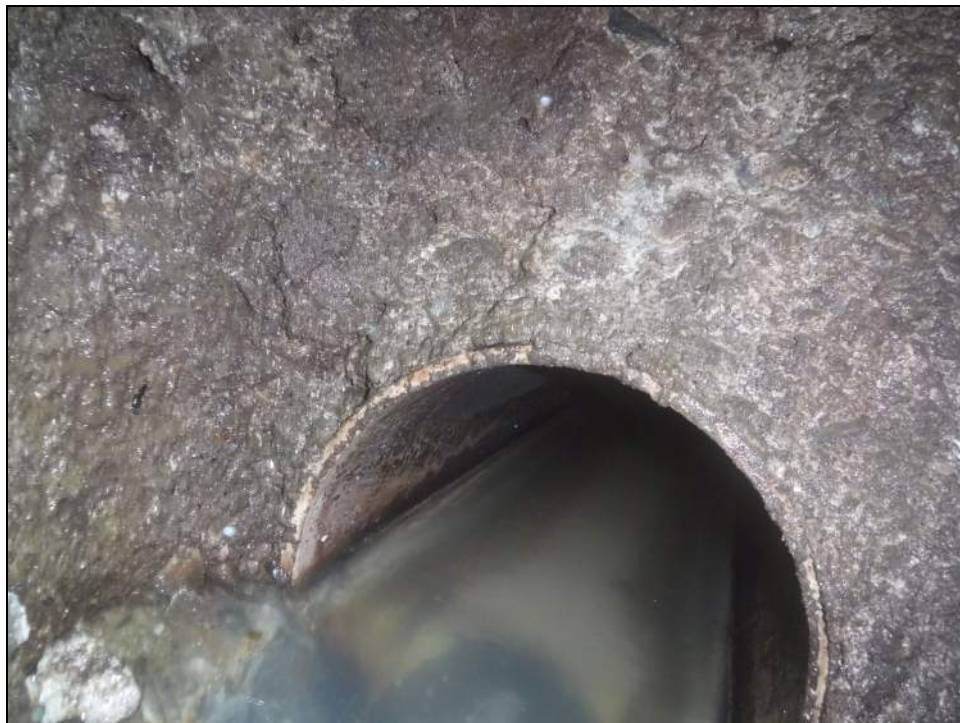
South Influent Pipe
