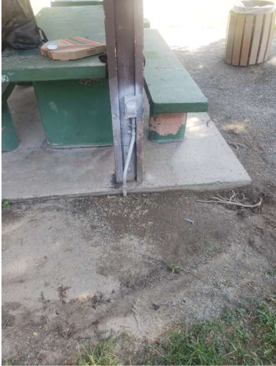
Arbor 3 – Electrical Outlet Location (view outside post)
