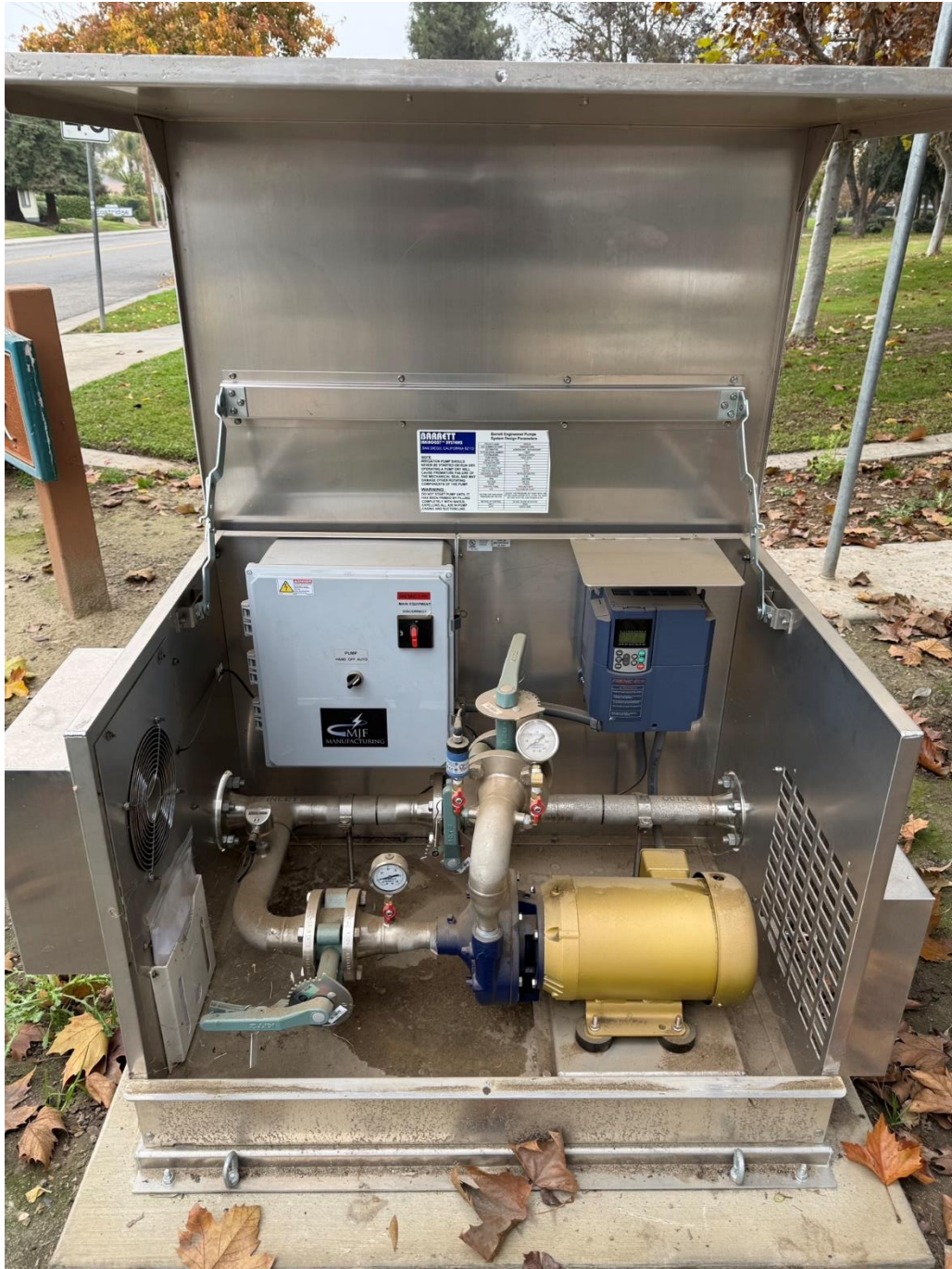
Figure 2 – New irrigation booster pump installed at Pinkham Park
