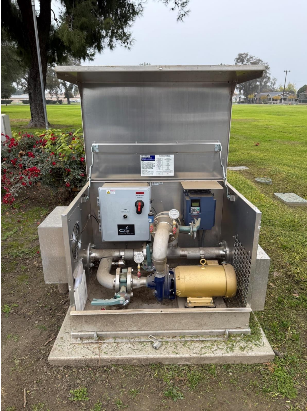
Figure 6 – New irrigation booster pump installed at Jefferson Park
