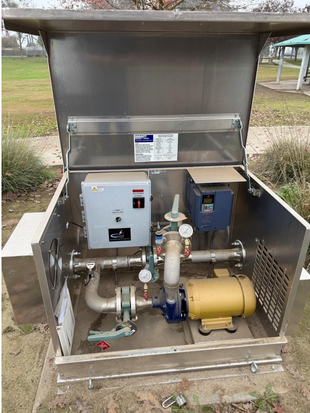
Figure 1 – New irrigation booster pump installed at Riverbend Park
