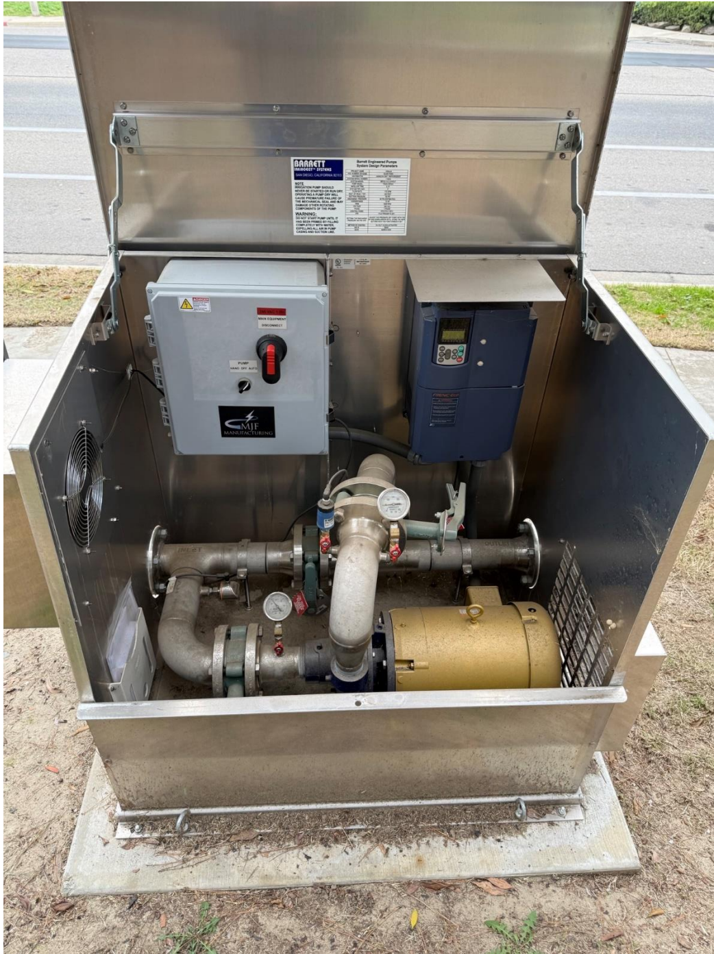
Figure 5 – New irrigation booster pump installed at Blain Park (Pump #2)
