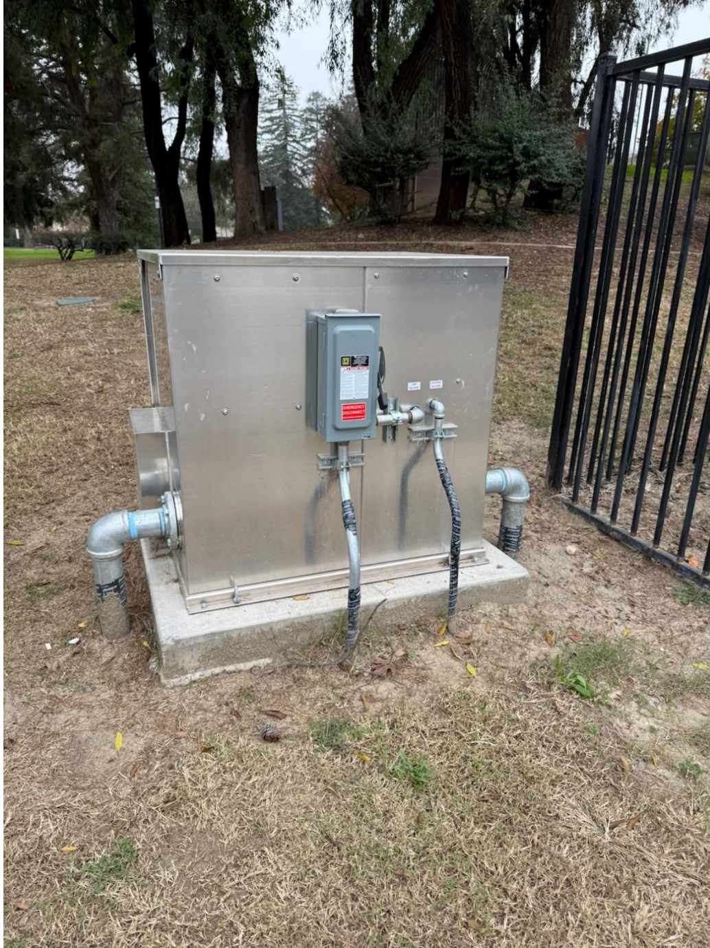
Figure 4 – New irrigation booster pump installed at Blain Park (Pump #1)
