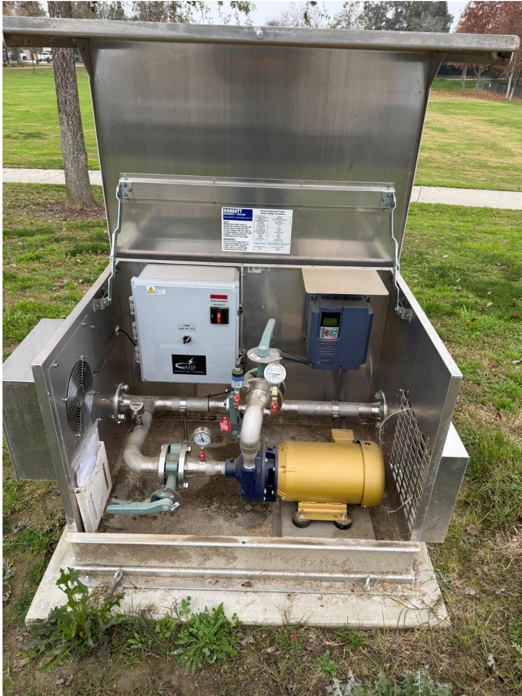
Figure 3 – New irrigation booster pump installed at Burke Park
