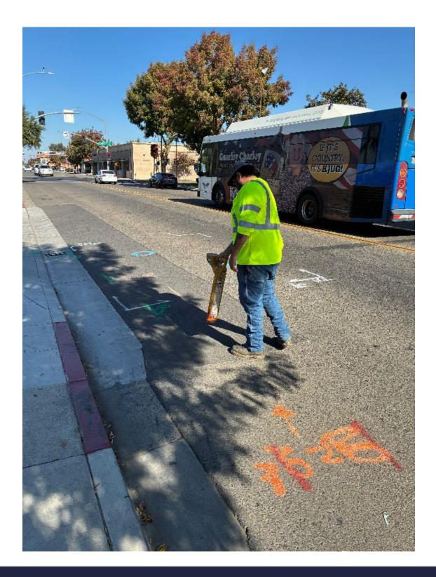
All of the city's underground infrastructure, including traffic signal, streetlight and fiber optic conduits, storm drain and sanitary sewer lines must be accurately located, marked, and documented. Everyday each (811) USA Dig ticket that comes through must be reviewed, marked out, and signed off to ensure protection of all city utilities during excavation.
