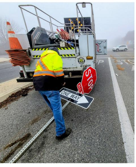
The city is divided into 14 sections for the blanket replacement of regulatory and street name signs. Each section is fully surveyed before placing an order for new signs. Once the order is received, installation and updates to the city's inventory log take several months to complete.
